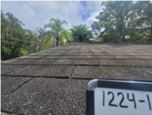
1224-1 Asphalt Shingle/Tar Typical Exterior Roof
