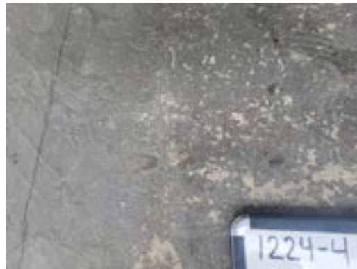
1224-4 Concrete Exterior Front Porch Floor
