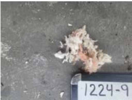
1224-9 Insulation Typical Interior
