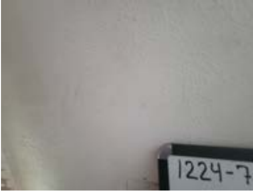
1224-7 Plaster Typical Interior Walls
