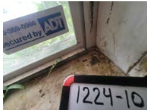
1224-10 Caulk Typical Interior Windows
